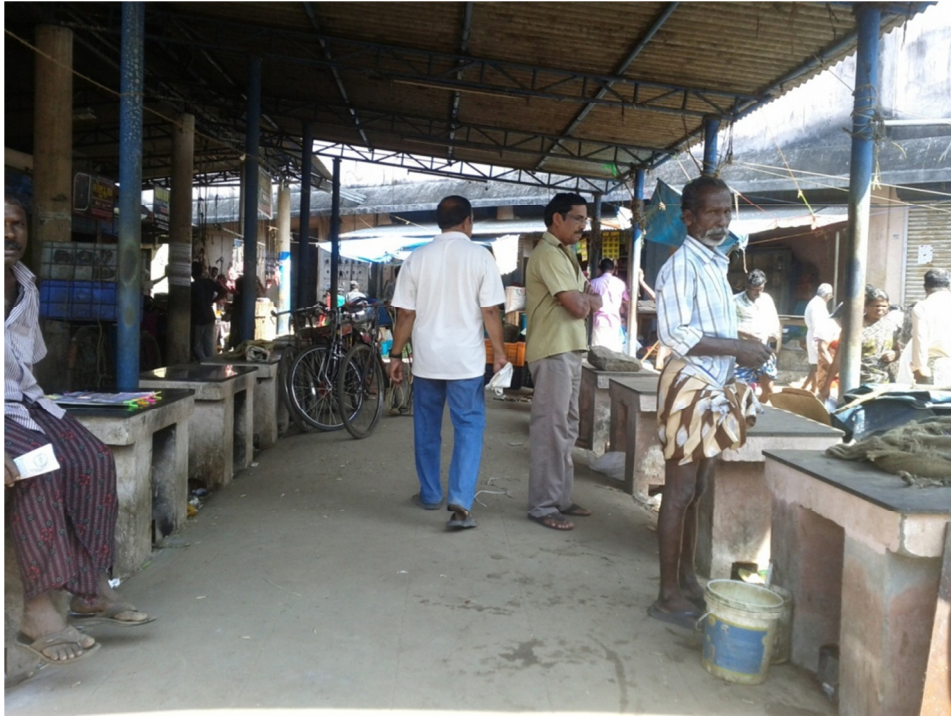
Ramankulangara fish market constructed for fish vendors(not is use)
