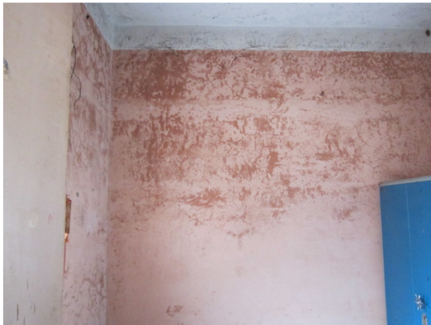
Roof Leakages due to poor water proofing of roof
