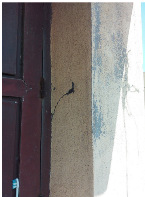
Cracks in the RCC Window Frames in Ernavur Kuppam
