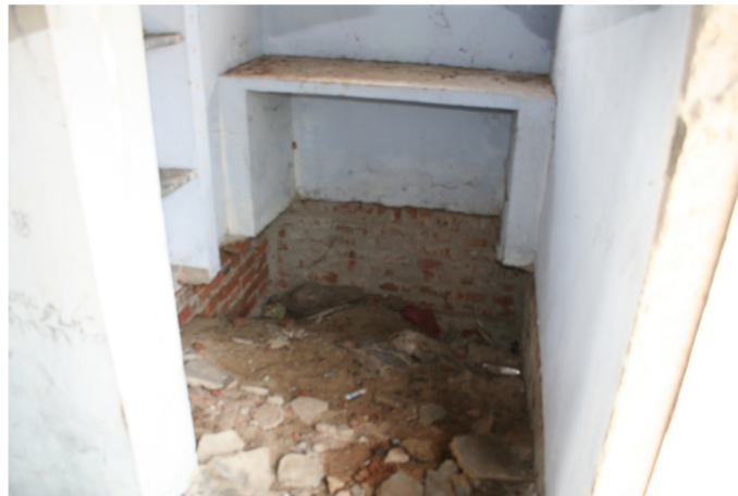
Collapse of Flooring due to Erosion in Kameswaram
