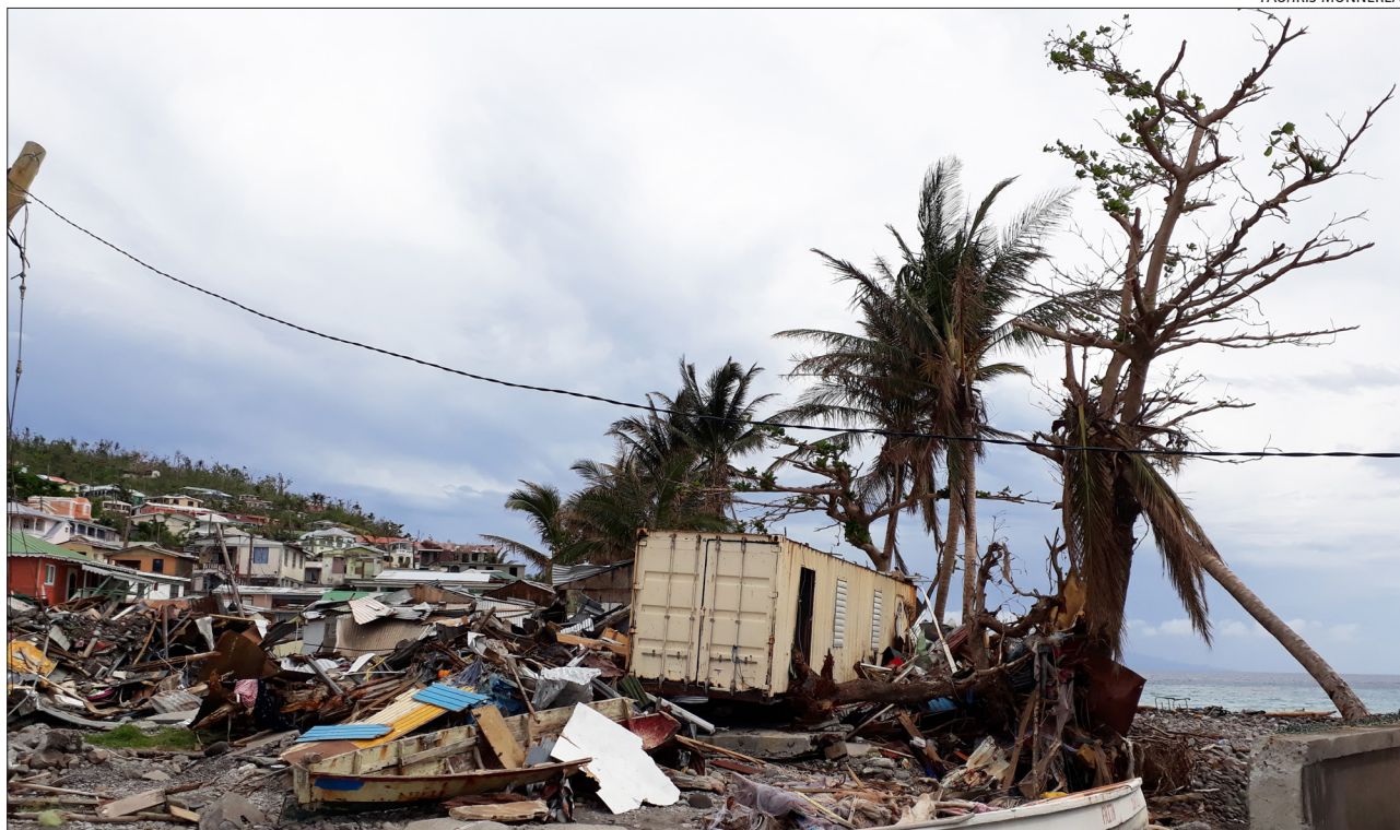
Hurricane Maria's damage in Scott's head, Dominica. In Dominica, hurricane Maria affected the basic livelihoods of approximately 2,200 fishers and fishworkers. The container is the fishing cooperative which was destroyed as a result of the hurricane
