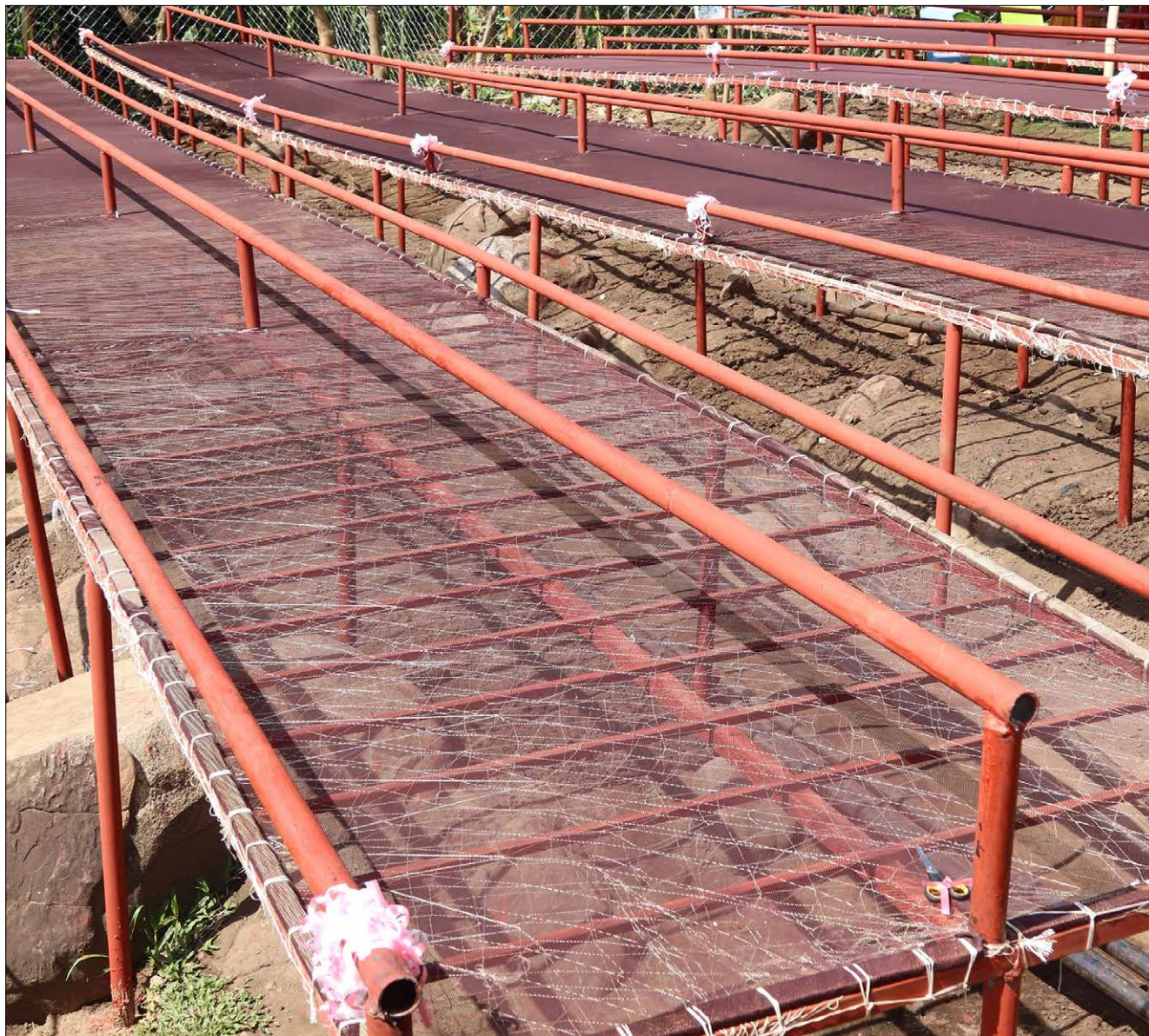
Modern drying racks made of steel, constructed to improve the processing of dagaa for women and sustain in the climatic shocks, Tanzania. By providing a reliable and sustainable means of drying dagaa , the racks have improved the overall resilience of the women's businesses
